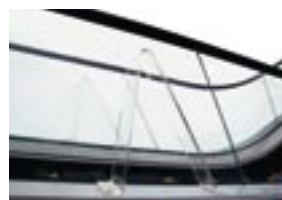
Anti climb barrier
