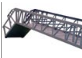
Hot dipped galvanised truss provides full corrosion protection
