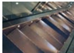
LED skirt lighting
